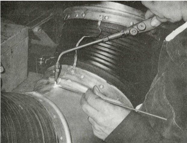
For repetition work other methods of pre-heating, such as air and gas torches etc, may be used. It is possible to speed up production by arranging procedures so that one or two assemblies are being pre-heated while others are being brazed.
